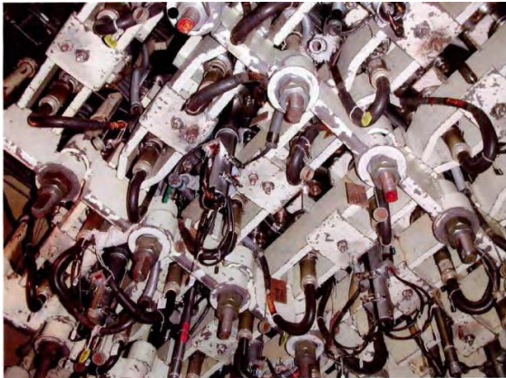
Status of CRD housing support before the Accident at Unit 3
